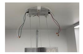
Pass suspension cables through grommets in canopy and lock into cable grippers in ceiling plates.
