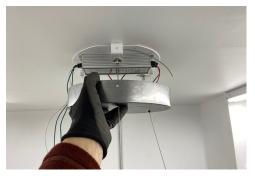
Slide the canopy up to meet the ceiling plate.
