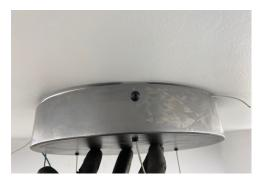
Fasten the Canopy in place with provided button head screws.
